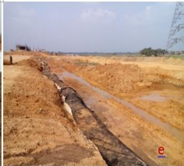
a) Laying of Coarse sand, b) Laying of Non-Woven Geo-textile, c) Laying of Granular Blanket. d) Laying of Woven Geo-textile, e & f) Stage construction of embankment.
