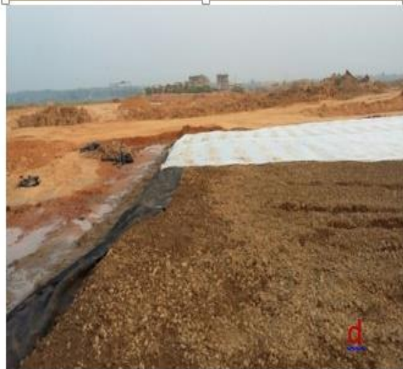
a) Laying of Coarse sand, b) Laying of Non-Woven Geo-textile, c) Laying of Granular Blanket. d) Laying of Woven Geo-textile, e & f) Stage construction of embankment.
