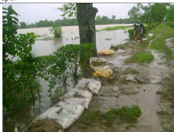
Fig. 5.4 Embankment protection by putting sand bags
