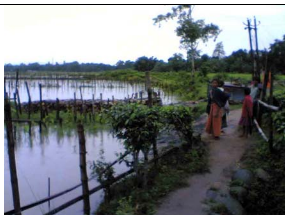
Fig. 5.2 Protection measure by putting bamboo spur
