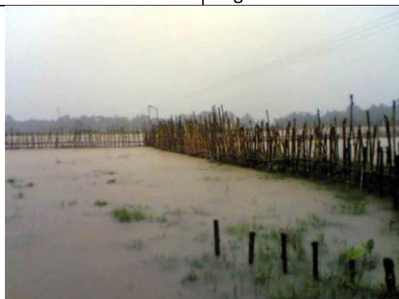
Fig. 5.5 Protection measure by using bamboo spur
