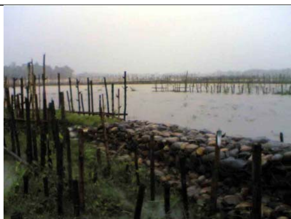
Fig.5.3 Embankment protection by using bamboo spur
