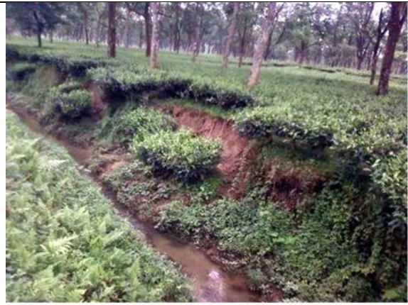
Fig. 4.6 Erosion in the main outlet drain
