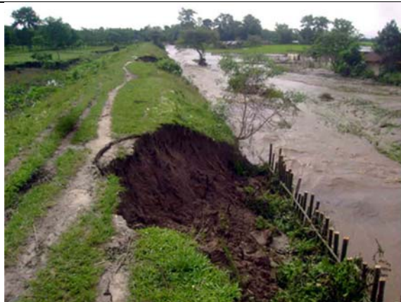
Fig. 4.5 Embankment failure due to erosion
