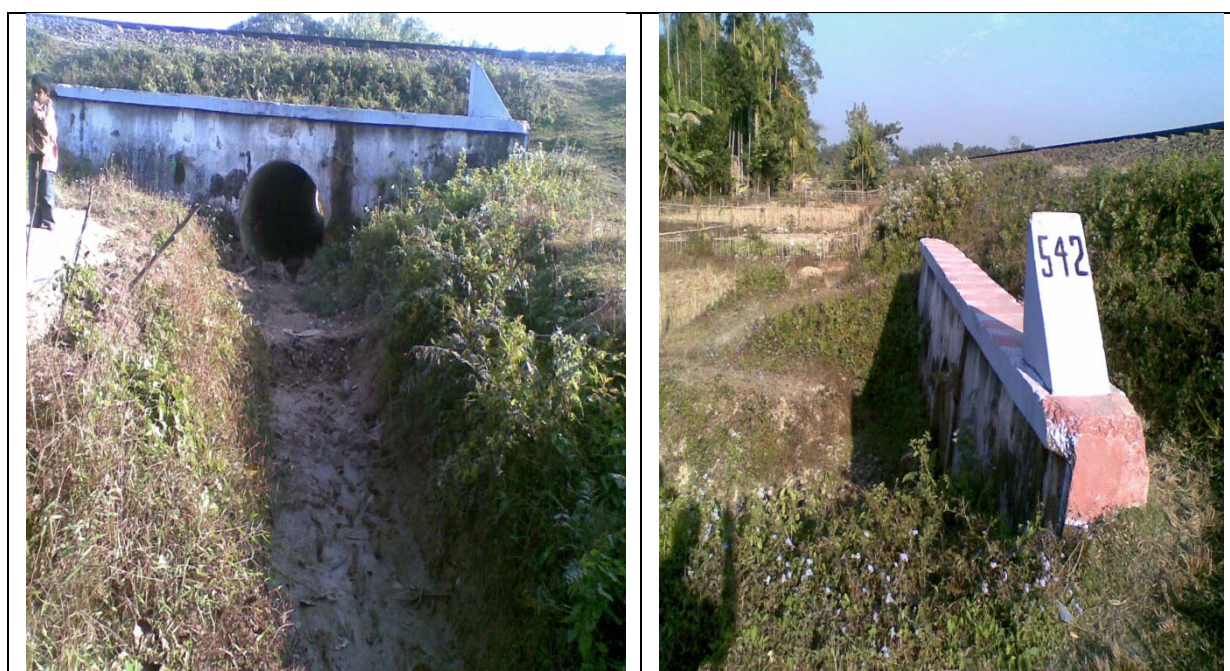
Fig. 4.9 Railway Culverts not carrying sufficient water
