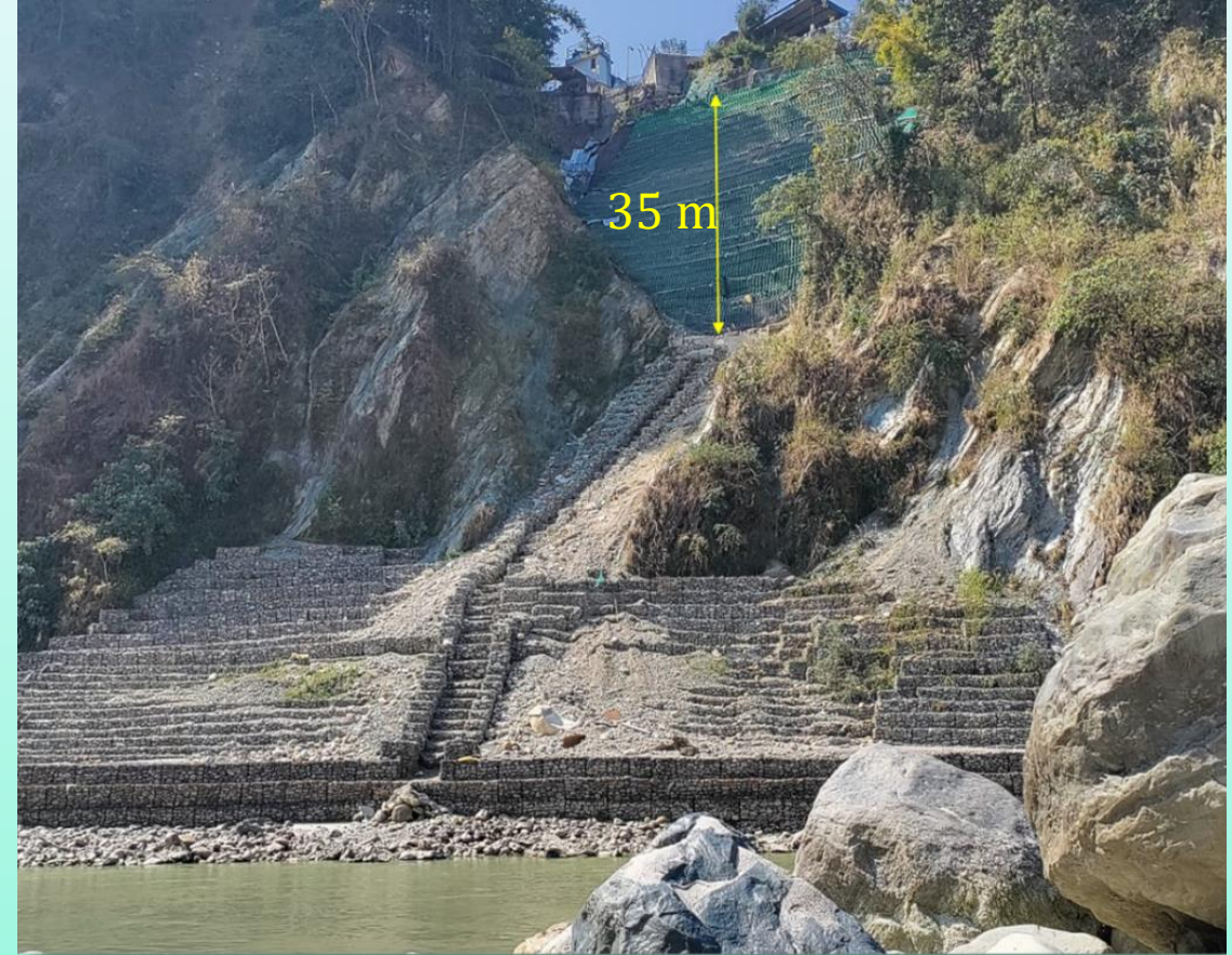
Gabion retention and GRS wall for reclamation
