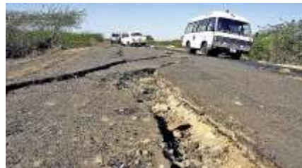
Fig 1. Road damage in Bhuj during 2001 Bhuj earthquake
