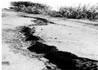
Fig. 2. Road damage at Chopadva during 2001 Bhuj earthquake
