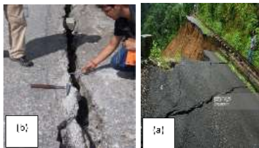
Fig. 3. (a) Ground rupture in Lachung as per Sharma et al., (2012); (b) collapsed portion of NH 55 between Siliguri and Darjeeling as per EERI (2012)
