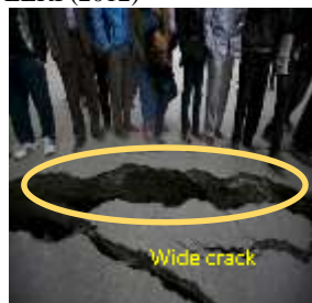
Fig. 4. Road cracks in Bhaktapur during 2015 Nepal earthquake as per Young (2015)
